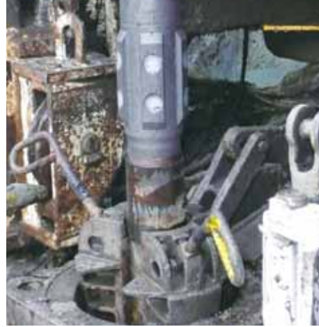
Far left: Applying pipe dope to BPS collar threads.
